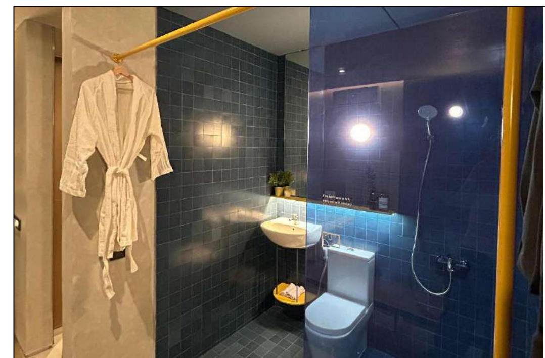
Interior Finishing for the Bathroom Area
