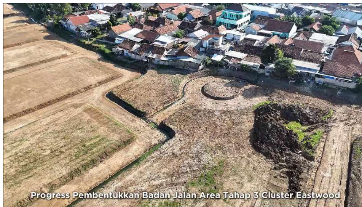
Phase 3 Eastwood Cluster - Road Formation Progress
