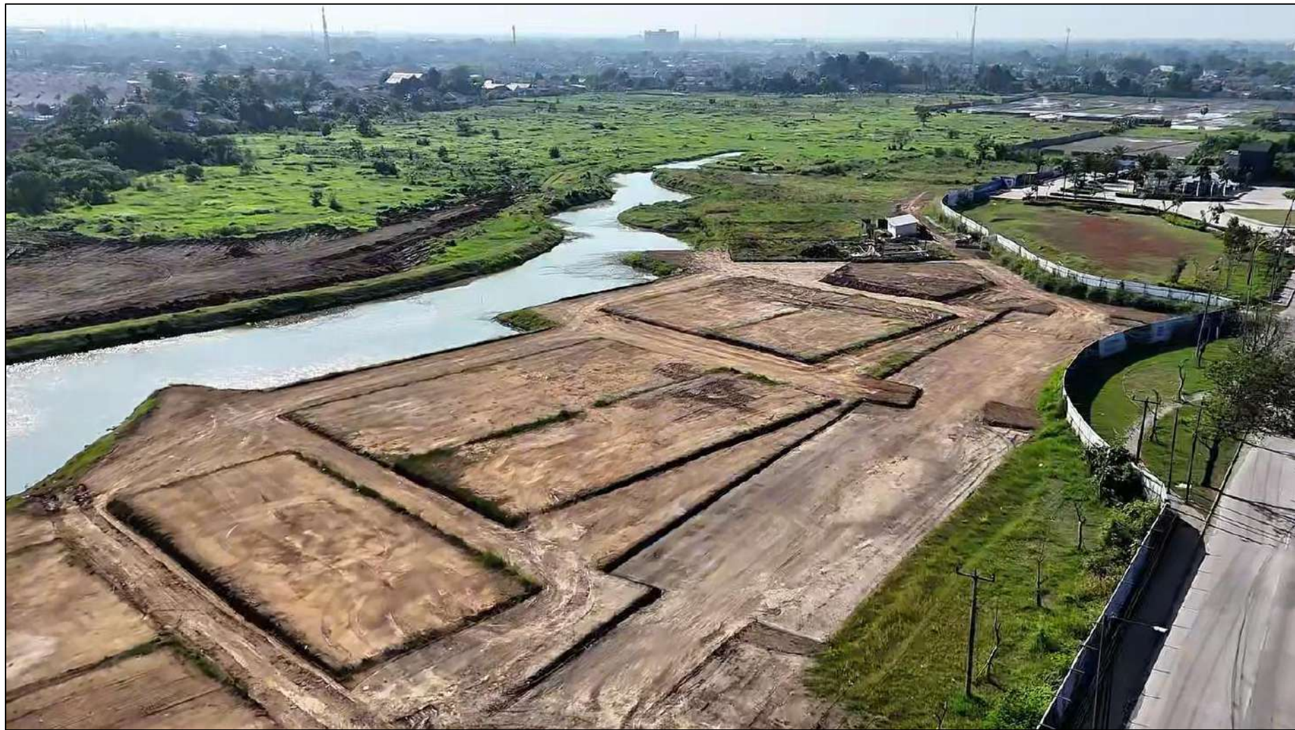
Commercial Shophouse Area - Land Cutting Progress
