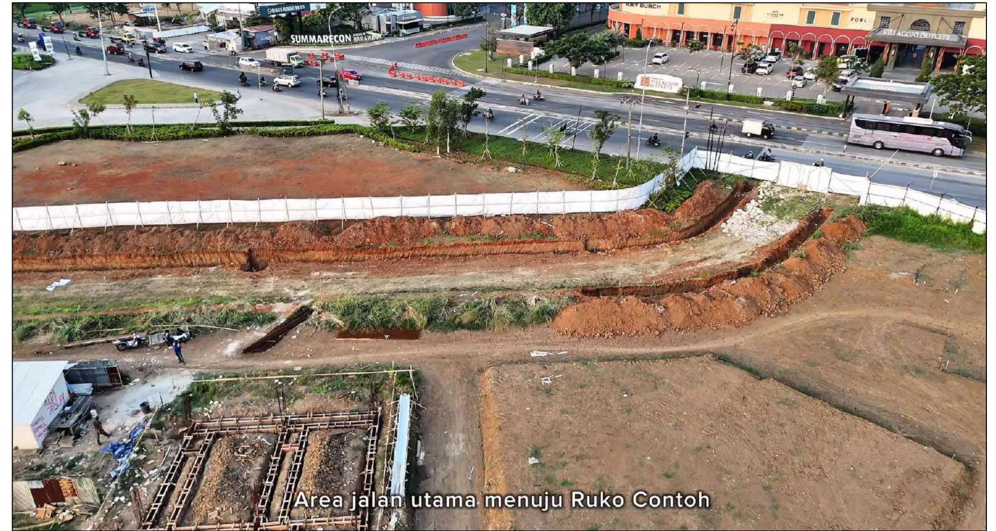
Commercial Shophouse - Road Formation Progress
