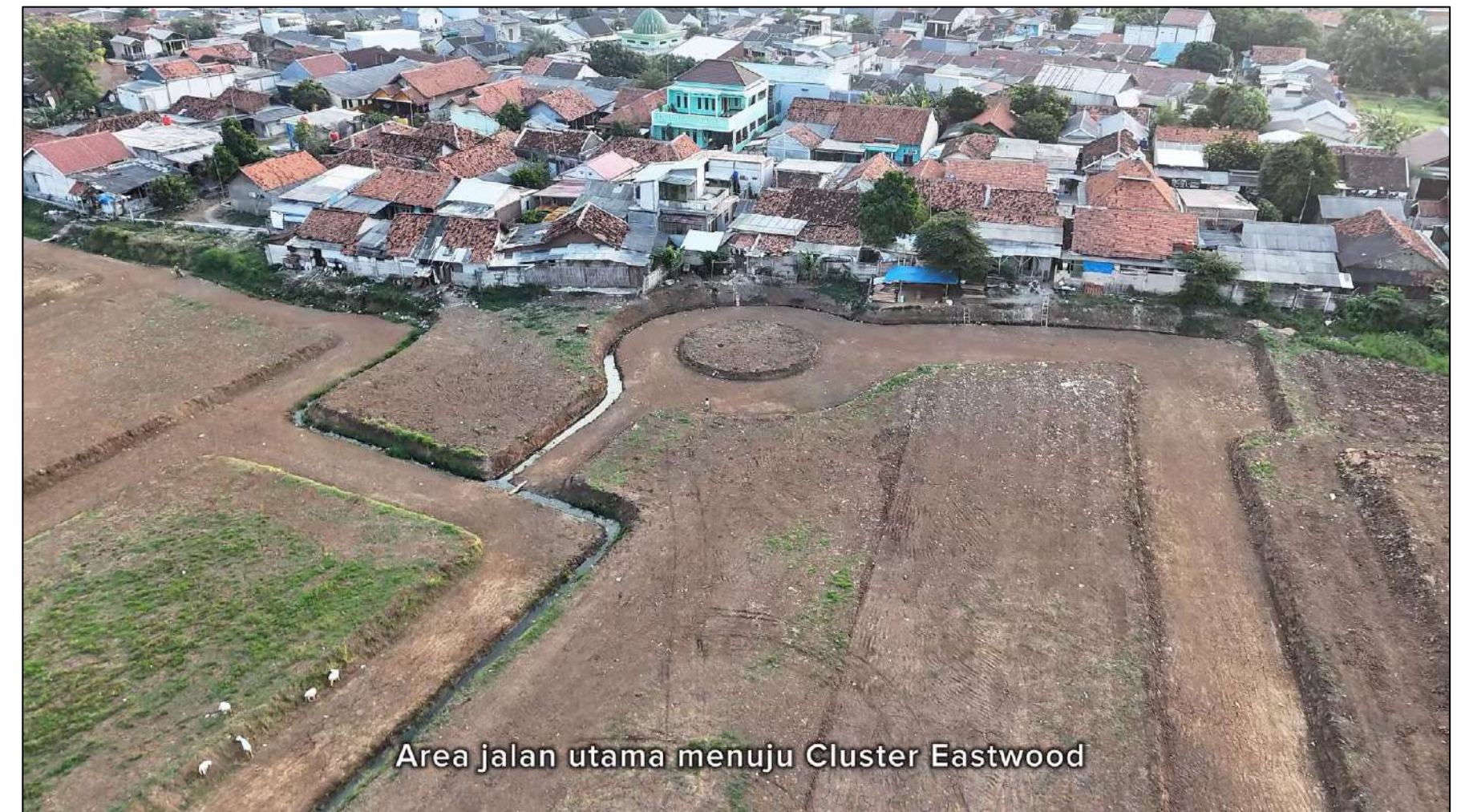
Eastwood Cluster - Road Formation Progress
