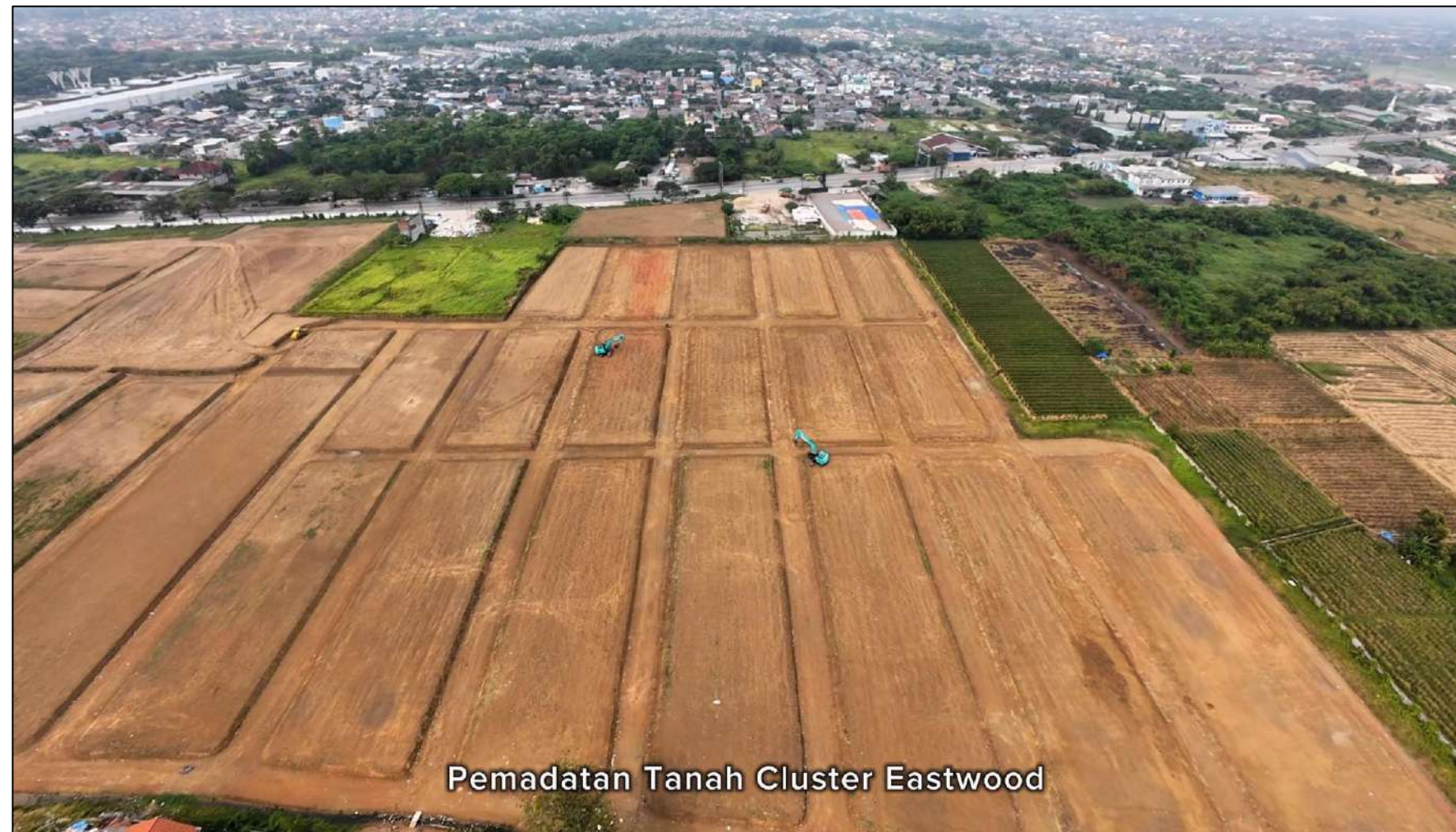
Eastwood Cluster - Land Cutting Progress
