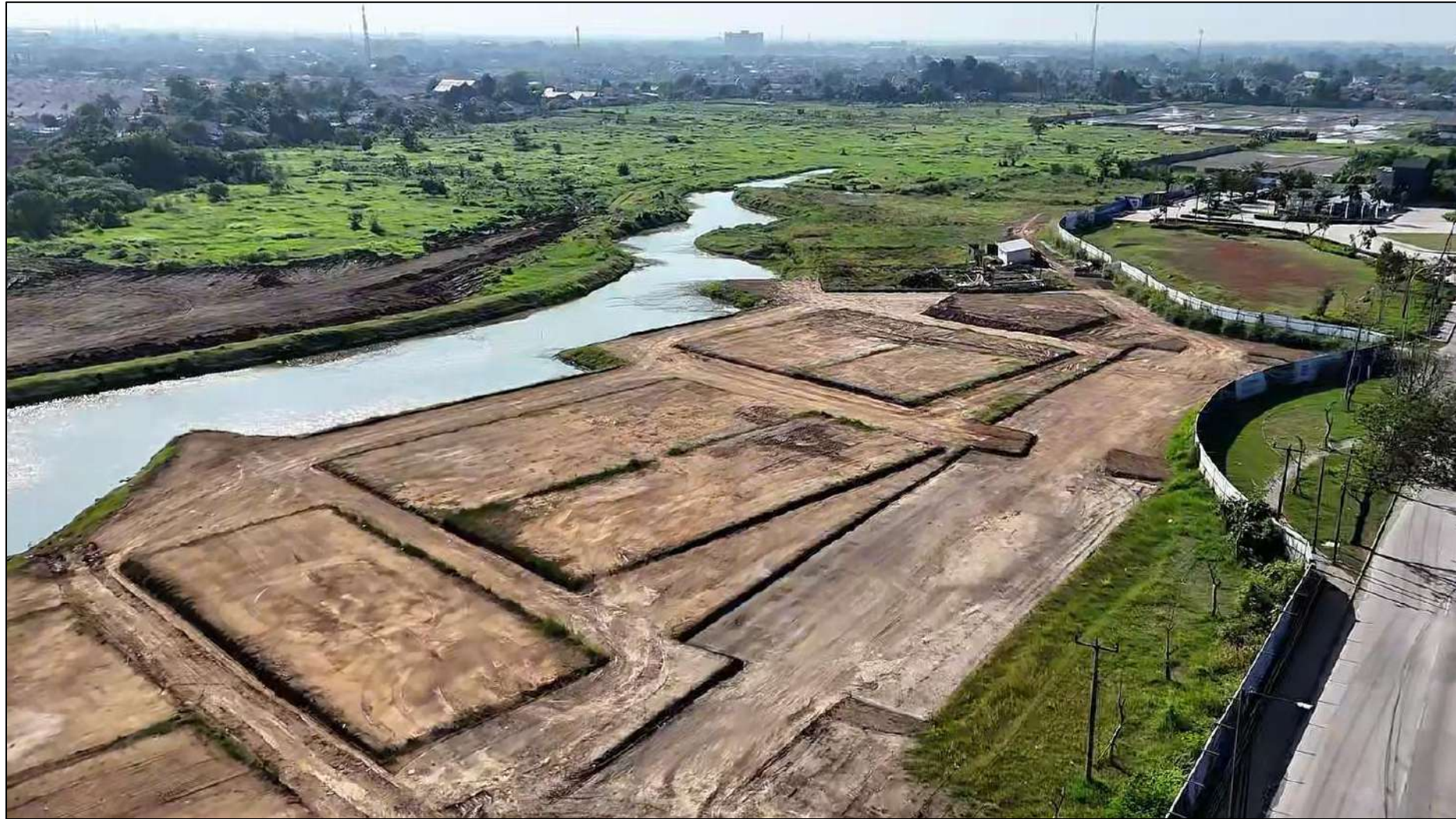
Commercial Shophouse Area - Land Cutting Progress
